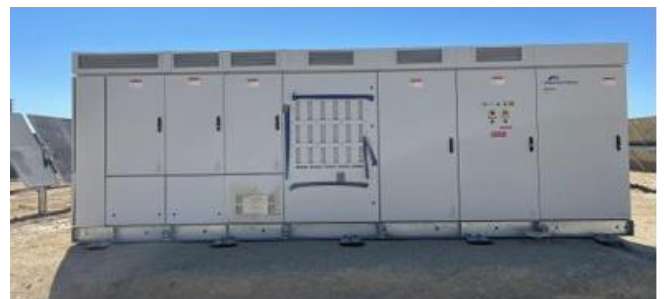
Example of a PCS without red safety chains installed:
